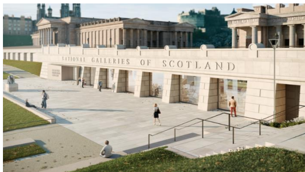
Scottish National Gallery, new entrance (Cadpeople & Hoskins Architects)
